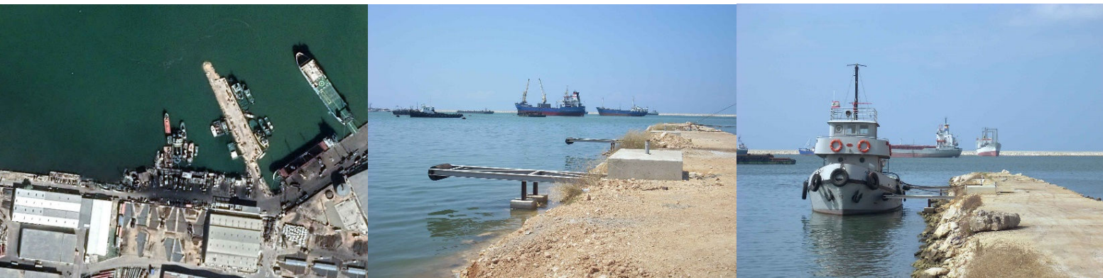
MOORING DOLPHINS AT TRIPOLI COMMERCIAL PORT
