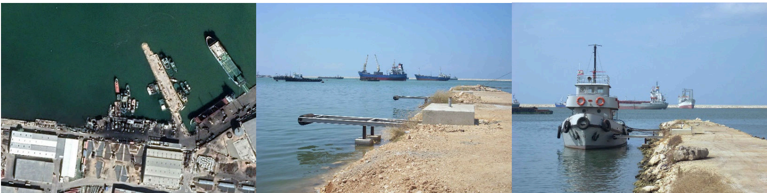
MOORING DOLPHINS AT TRIPOLI COMMERCIAL PORT
