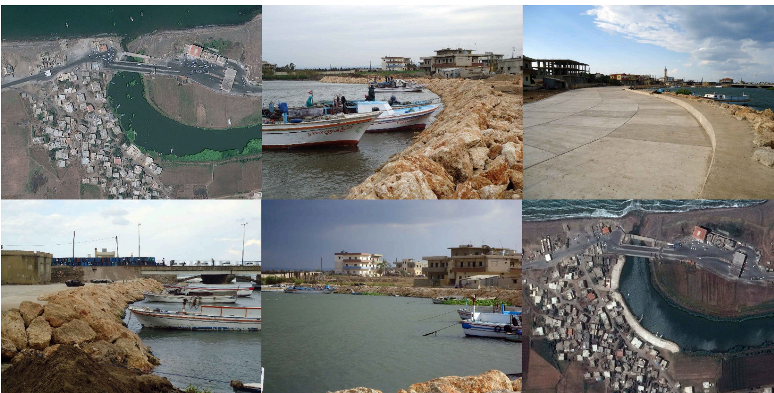
PROTECTION OF NAHER EL KEBIR RIVER BANKS
