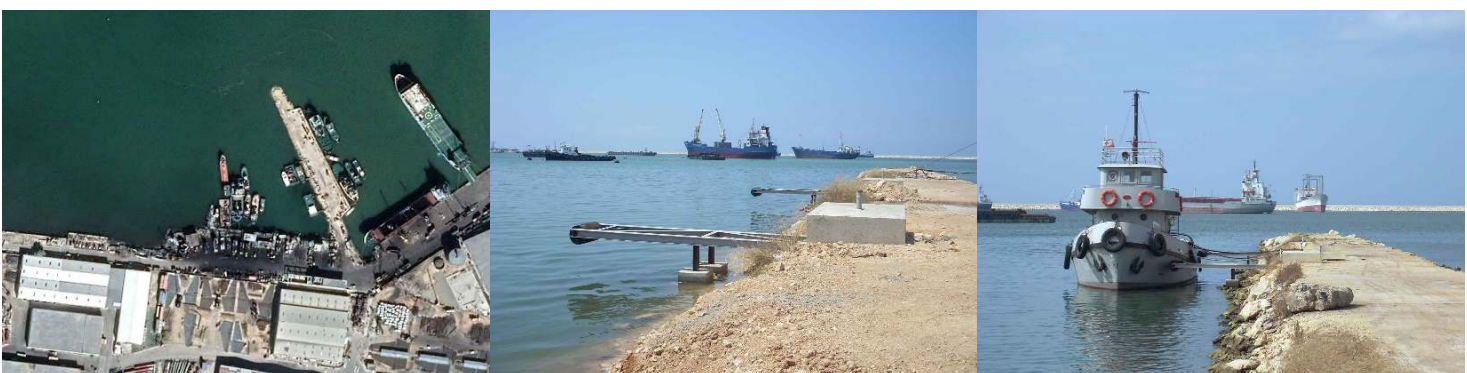
MOORING DOLPHINS AT TRIPOLI COMMERCIAL PORT
