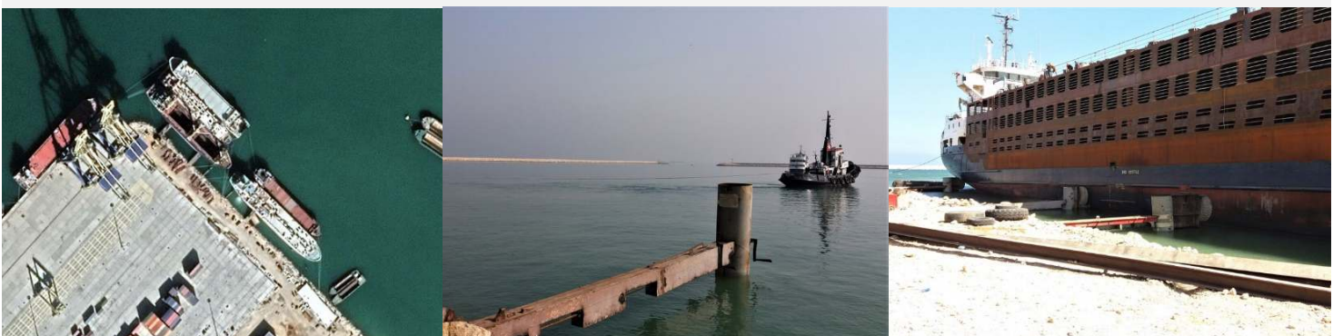
MOORING PILES AT TRIPOLI COMMERCIAL PORT
